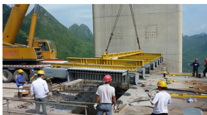
One of the TENSA®MODULAR expansion joints during installation
