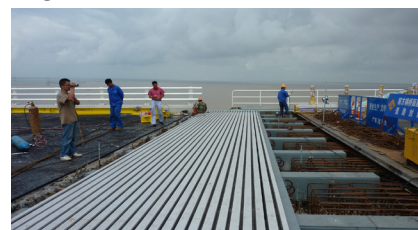
An expansion joint after positioning in the bridge deck
