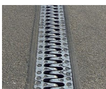
Cantilever finger joint
