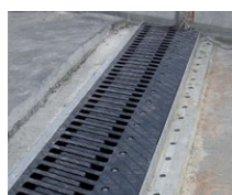
Sliding finger joints
