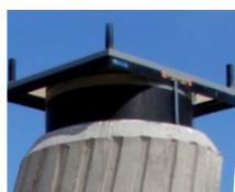
Deformation bearings
