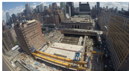
Construction site with railway tracks to Penn Station being covered by the huge box girders
