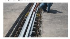
An installed TENSA®GRIP RS joint, with hump seal and ROBO®DUR asphalt reinforcing ribs
