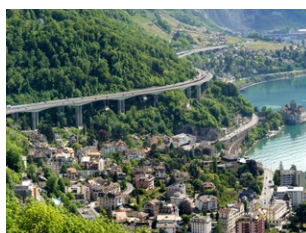
Viaduct de Chillon, Switzerland
