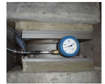
Lifting and measuring bearing
