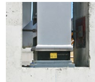
Reinforced elastomeric bearing
