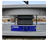
Pendulum bearing
