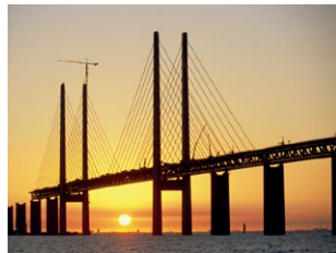
Öresund Bridge, Denmark
