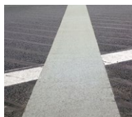
Flexible plug joint
