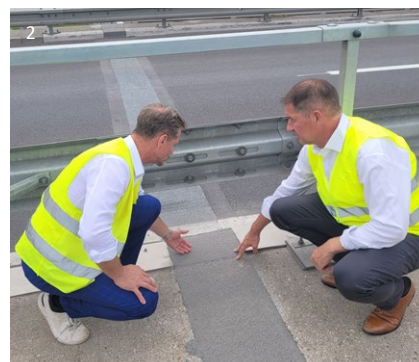
Sliding finger joint
