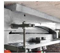
Cylinder bearing
