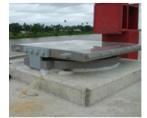
Incremental launch (ILM) bearing
