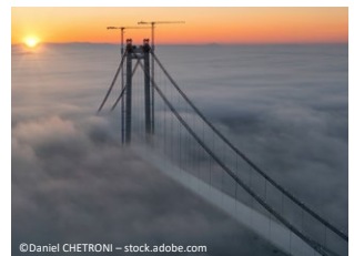
Braila Bridge, Romania
