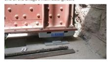
Two RESTON®STU shock transmission units during installation at one end of the bridge deck
