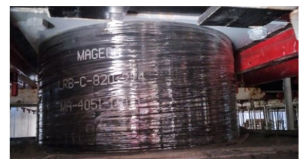
A LASTO®LRB lead rubber bearing in its final position
