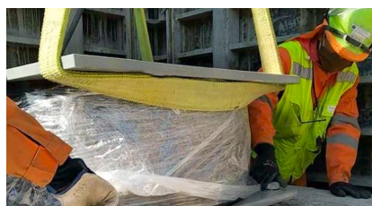
Installation of a LASTO®LRB isolator
