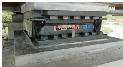
The installed spherical bearings are also equipped with dust skirts
