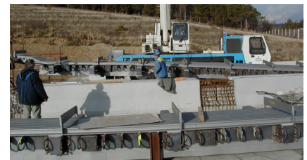
Installation of mageba LR9 expansion joints
