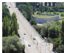
Pont Europe (CH)
