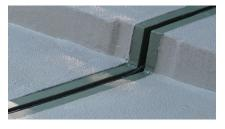
The joint's robust design and strong anchorages make it very durable, even under heavy traffic
