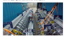
Installation of a TENSA®GRIP single gap expansion joint with sinus plates on the viaduct
