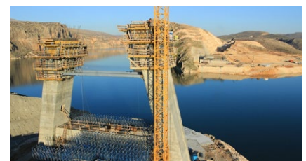
The bridge's piers under construction
