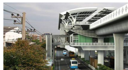
The Puchao Saming Phrai station after construction
