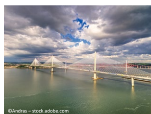
Queensferry Crossing, UK
