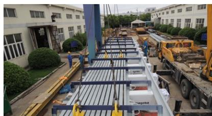
A TENSA®MODULAR expansion joint at one end of the cable suspended structure
