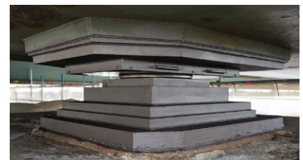
A new spherical bearing after installation
