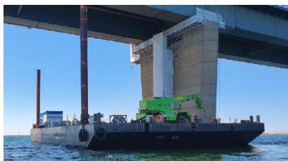
Fixed pontoon at the bridge's pier
