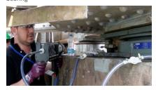
One of the pot type bearings after installation
