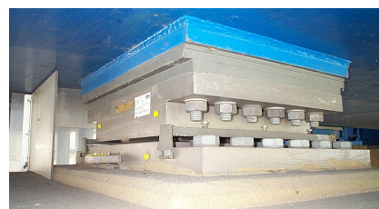
Installed horizontal force bearing
