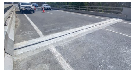
Installed TENSA®GRIP expansion joint on the Spirit of Progress Bridge
