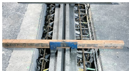
A TENSA®GRIP expansion joint during installation
