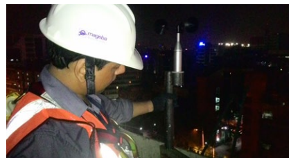
Night-installation of a wind sensor
