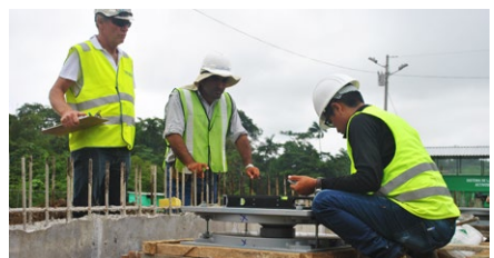
Precise positioning and levelling of a RESTON®PENDULUM seismic isolator
