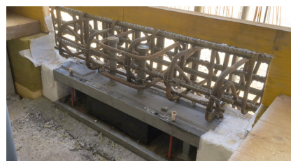
LASTO®BLOCK C before concreting with steel bars
