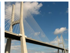
Vasco da Gama Bridge (PT)
