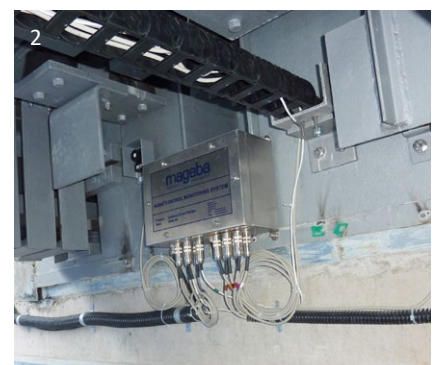
1 Installation of exceptional TENSA®MODULAR LR24 expansion joint 2 ROBO®CONTROL box as installed
