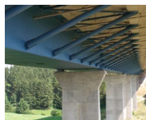
Steinbachtal Bridge (DE)
