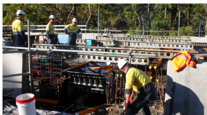
The mageba TENSA®MODULAR expansion joint during installation on the first viaduct
