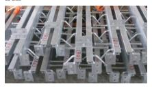
An expansion joint as installed, showing its "concrete connection" at surface level
