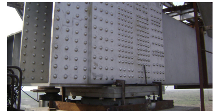
A RESTON®POT bearing as installed, during erection of the bridge deck on top of it.
