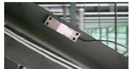
Strain measurement on one of the bridge deck's steel members
