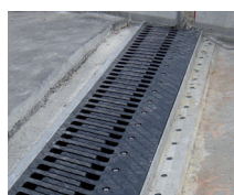
Sliding finger joints
