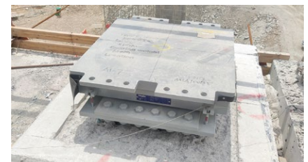
A RESTON®SPHERICAL bearing installed on site
