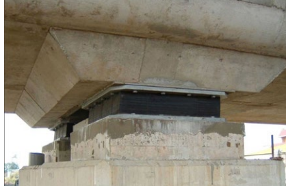
Lead rubber bearings
