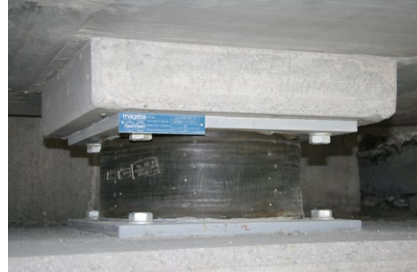
High damping rubber bearings
