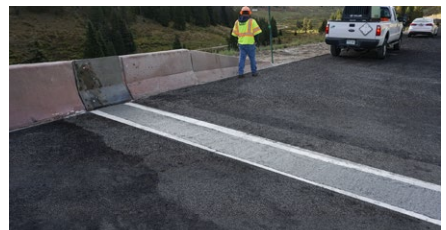
The completed flexible plug expansion joint high in the Rocky Mountains of Colorado
