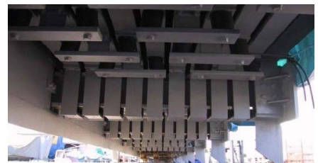
View of a modular expansion joint from beneath, showing its control mechanisms
