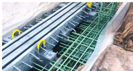
TENSA®MODULAR LR3 joint is being installed
