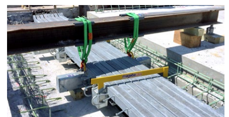
Modular joint installation
