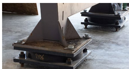
View of the LRBs following installation to support the anaerobic digester
