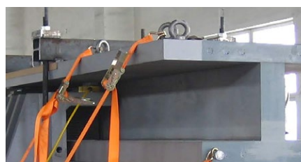
Preparing the special bearings for transport
