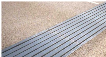
A modular expansion joint of the type required by the new bridge
