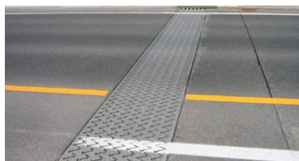
A modular expansion joint featuring noise-reducing "sinus plates" on its surface
