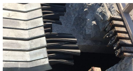
New mageba expansion joint next to existing joint to be replaced
