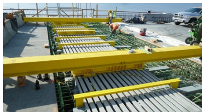
Installation of a 16-gap TENSA®MODULAR LR joint
