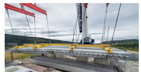
Finger joint is lowered into the bridge deck block out
