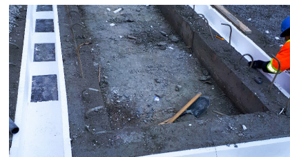
Installed VIBRAX®BLOCK B elastomeric bearings
