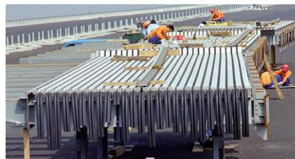
View of the underside of a TENSA®MODULAR joint of type LR27, prior to installation
