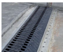
Sliding finger joints
