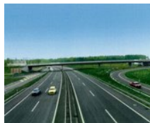
Freeway overpass Moosgasse, (CH)
