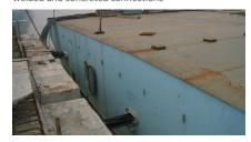
Due to their great size, the TENSA® MODULAR expansion joints were assembled on site
