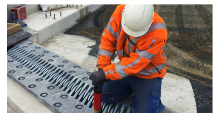
A TENSA®FINGER RSFD cantilever finger expansion joint during installation on site
