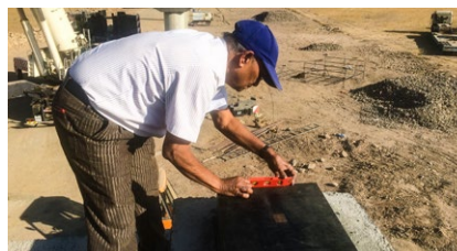
Installation supervision of LASTO®BLOCK elastomeric bearings
