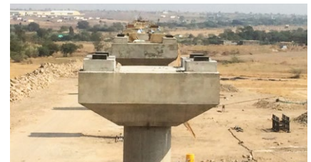
Installed LASTO®BLOCK bearings pairs on top of the bridge's pylons
