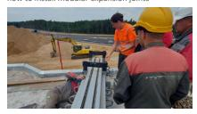
Installation of mageba's ROBO®STATIFLEX reinforcing beam next to a joints
