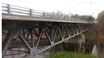
The bridge over the Roeliff Jansen Kill river
