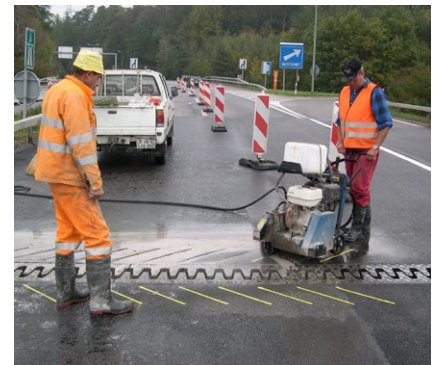
Cutting of slits at a 45° angle to the driving direction
