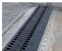
Sliding finger joints
