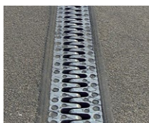
Cantilever finger joint
