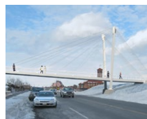
Revere Bridge (US)
