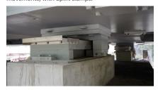
A TENSA®MODULAR joint (type LR3) during installation at one end of the bridge's deck.
