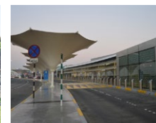
Abu Dhabi Airport (UAE)
