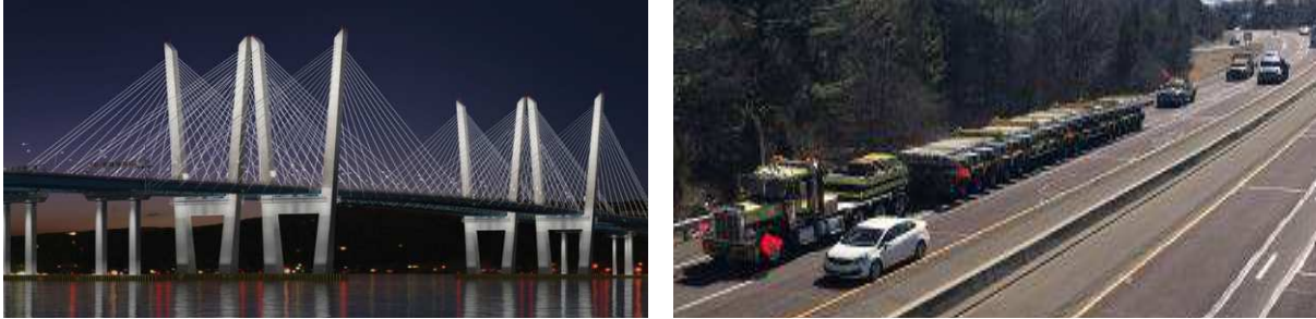
Figure 7. The new Tappan Zee Bridge (left), and road transport to site with police escort (right)
