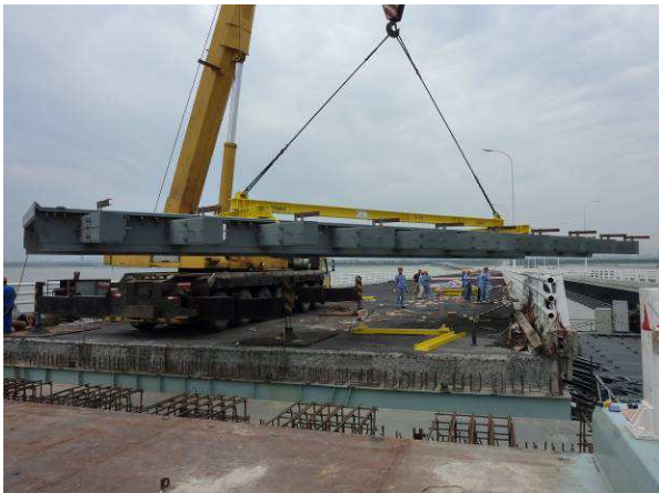
Figure 6. Lifting in and installation of a 22-gap modular joint on the Chongming Bridge, 2008
