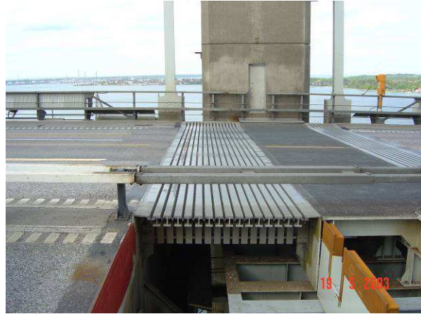
Figure 11. Installation of 7-gap and 14-gap Tensa-Modular expansion joints, side by side, during renovation of the Lillebaelt Bridge, Denmark (2002)
