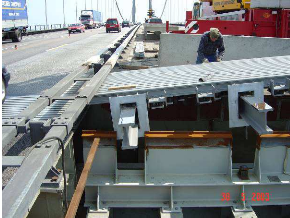
Figure 11. Installation of 7-gap and 14-gap Tensa-Modular expansion joints, side by side, during renovation of the Lillebaelt Bridge, Denmark (2002)
