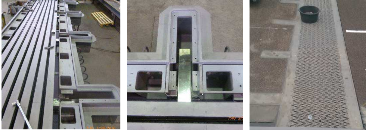
Figure 14. A Tensa-Modular expansion joint as specially designed for easy future renewal by means of the “Quick-Ex” method – maintaining the joint’s connections to the main structure
