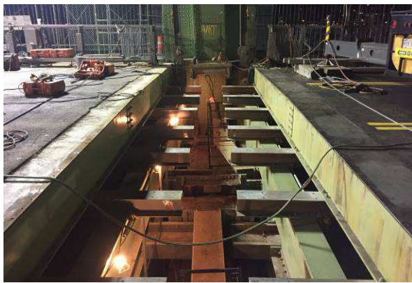
Figure 12. Installation of a 7-gap Tensa-Modular expansion joint during renovation of the Angus L. Macdonald Bridge in Halifax, Canada (2017)
