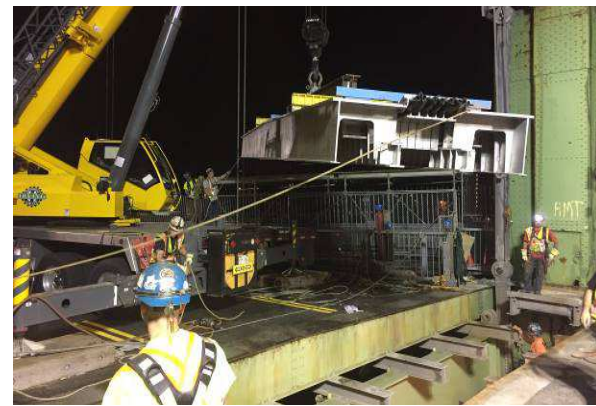
Figure 12. Installation of a 7-gap Tensa-Modular expansion joint during renovation of the Angus L. Macdonald Bridge in Halifax, Canada (2017)
