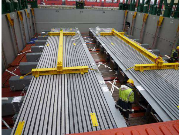
Figure 2. Two 24-gap Tensa-Modular joints being secured in a ship's hull for transport to site (left), and one of these during lifting into position on site (right)
