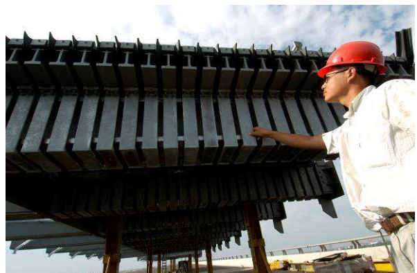
Figure 3. The Run Yang Bridge in China (left), and one of its 27-gap modular joints on site (2005)
