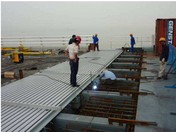
Figure 6. Lifting in and installation of a 22-gap modular joint on the Chongming Bridge, 2008
