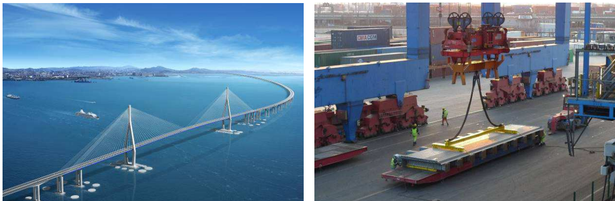
Figure 1. The Incheon Bridge (left), and one of its 24-gap joints during loading onto a ship (right)
