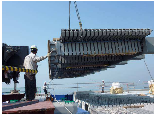
Figure 2. Two 24-gap Tensa-Modular joints being secured in a ship's hull for transport to site (left), and one of these during lifting into position on site (right)
