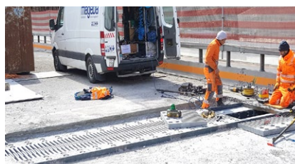
A TENSA®FINGER GF joint during installation
