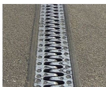
Cantilever finger joint
